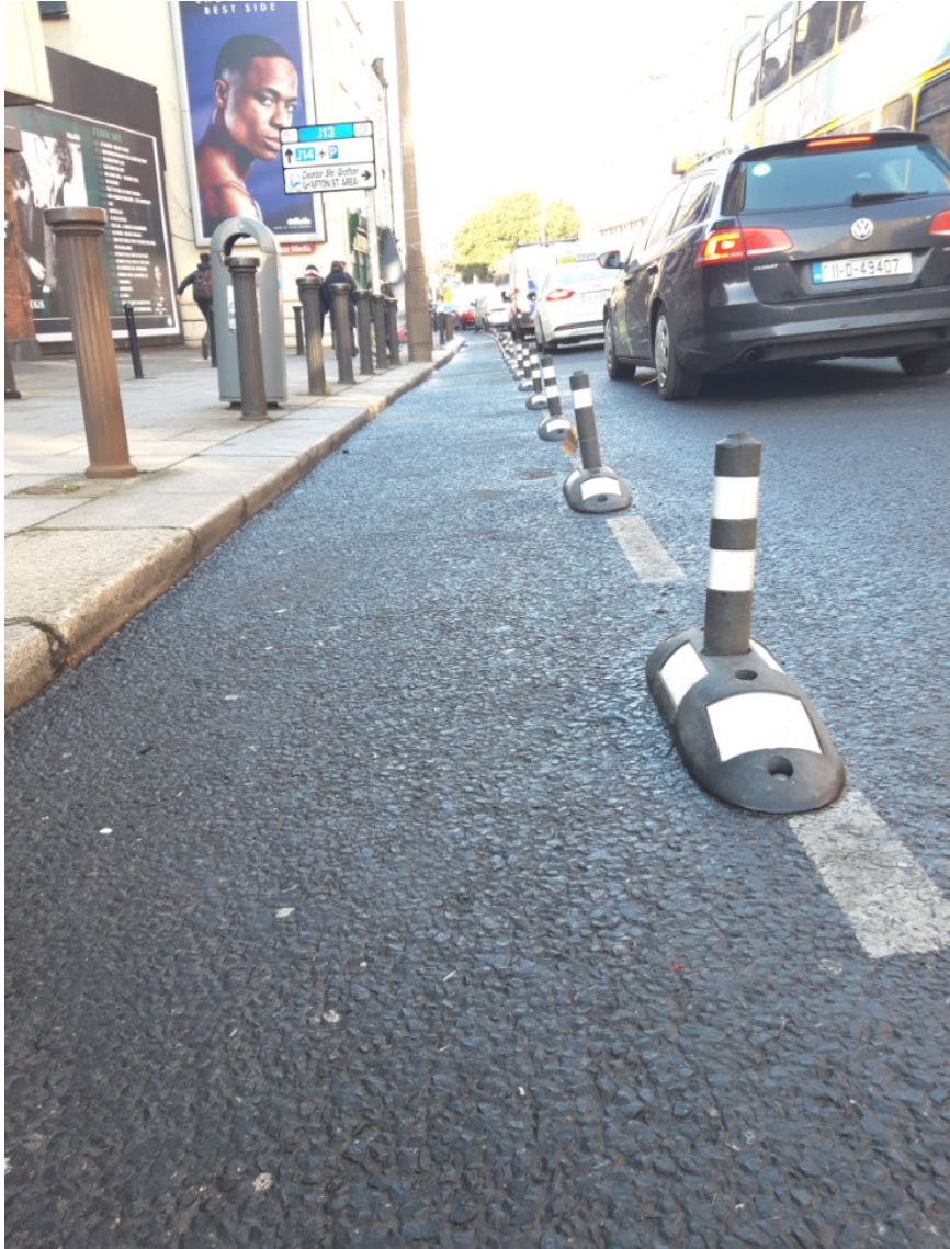
Fig 1.1- Photo of Lane Separators (Orcas) between the cycle lane and the traffic lane on Leeson Street.
